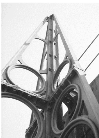
One of the cast iron triangular guides of the 1830 No 2 Gasholder, seen here in 1972; a security fence currently prevents close access.
