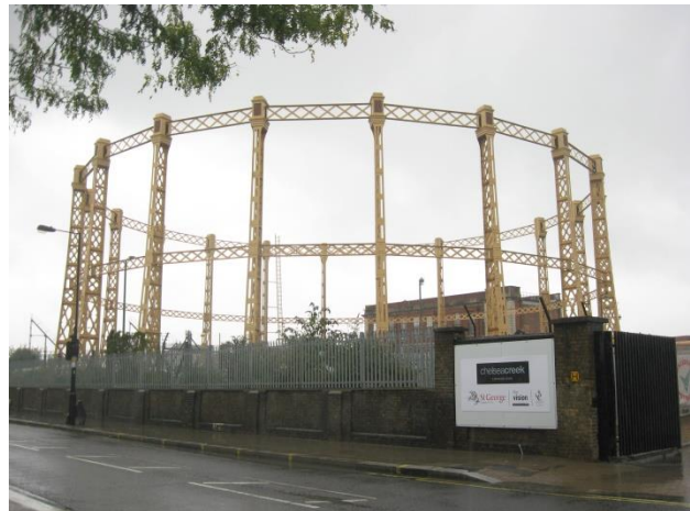
The elegant cast and wrought iron guide frame of No 7 Gasholder, part of which we hope can be incorporated in the site redevelopment.
