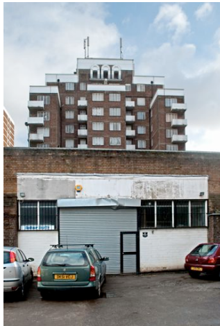
This garage under Shepherd's Bush Road (with The Grampians in the background) was once a tunnel carrying the L&SWR commuter line between Richmond and Waterloo.
