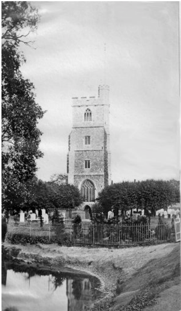
A splendid view of the medieval tower of All Saints Church, Fulham, taken in 1874, showing the palace moat in the foreground. The tower is threatened by the heavy church bells knocking against it when rung – see update right.
