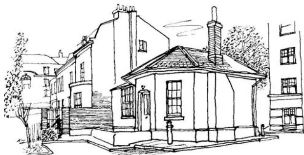
The listed cottage adjacent to early 19th century Temple Lodge in Queen Caroline Street, recently restored as part of the St Vincent's care home rebuilding.
