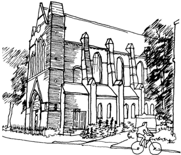
Holy Innocents, Paddenswick Road, designed by James Brooks and consecrated in 1891. The west wing was added in 1901.
