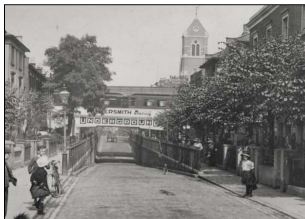
This 1905 photograph of Cambridge Grove clearly shows the railings either side of the roadway which has been lowered to pass under the railway bridge. The tower of St John's church (see page 2 above) stands in the background.
